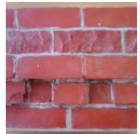
Photo: Reflex Section of fibreglass replica chimney
