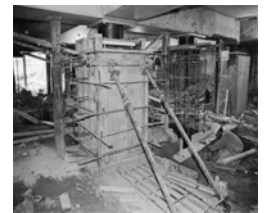
Installation of base isolators at Parliament Buildings, 1993
