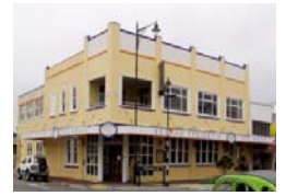
Speights Ale House, Jackson Street, Petone Registered Historic Area Earthquake strengthened, 2004 Photo, Havill Building LTd
