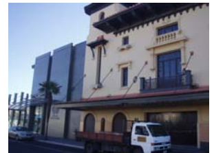
Hastings Municipal Theatre, Hastings, registered Category I historic place. The addition was constructed in 2005 to enable improved use and access into the theatre while preserving interior fabric. Photo, NZHPT 2007
