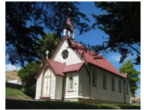
St Josephs Church, Pauatahanui, registered Category I historic place. As part of restoration works in 2004, a new driveway was built to improve access to the church. Photo, NZHPT 2007
