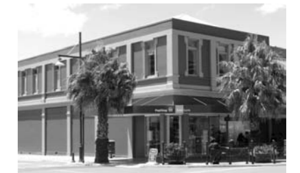
Looks can be deceiving when it comes to earthquake damage. Rosie's building did not show outward signs of significant damage to its street façades, but the brick walls were in bad shape – virtually to the point of collapse under the stress of the shake – some needing rebuild and others repair and strengthening. Photos left to right: after the earthquake (A Walters, Nicoll Blackburne Architects); essential rebuilding underway (G Henry, NZHPT), and completed (B Haynes, McCann 'ics).
