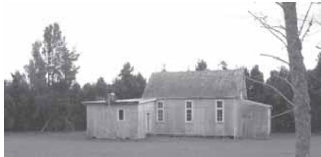
When maintenance became too costly the building was clad in asbestos boards whilst the shingle roof is believed to have been replaced with iron at quite an early stage. Photo: K Hearle, May 2006.
