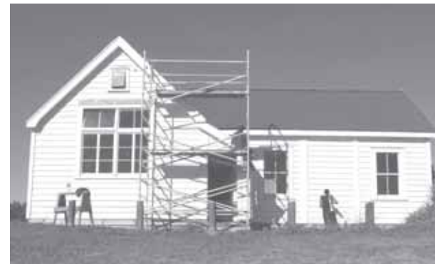
Priming the exterior of Te Kotukutuku School House. Photo: E Anderson, 2008.
