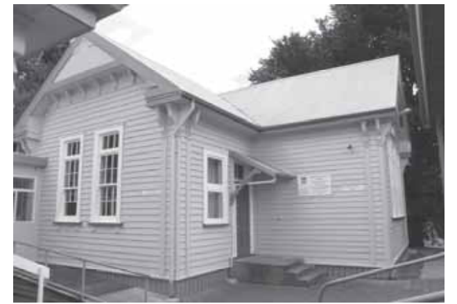
Te Kuiti School (Old Building). Photo: G Henry, 2010.
