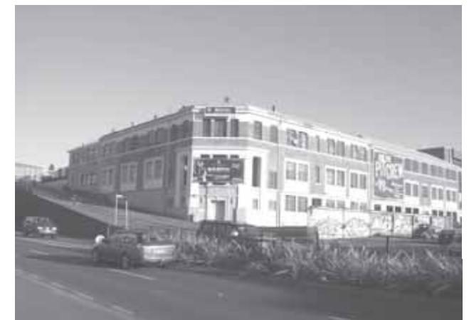
Waikato Institute of Technology (WINTec) F Block following its seismic strengthening, restoration and sympathetic changes to the entranceway and fenestrations, enabling the Block to continue its educational purpose. Photo: M Vincent, 2009.
