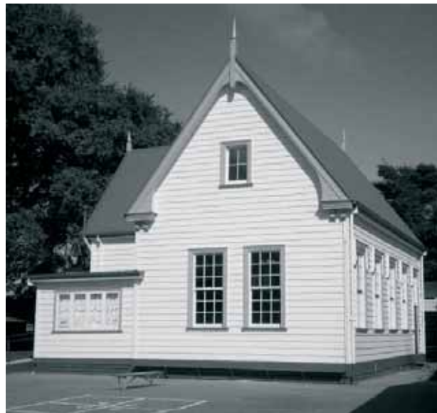
Tamahere School Original Building. Photo: L Williams.
